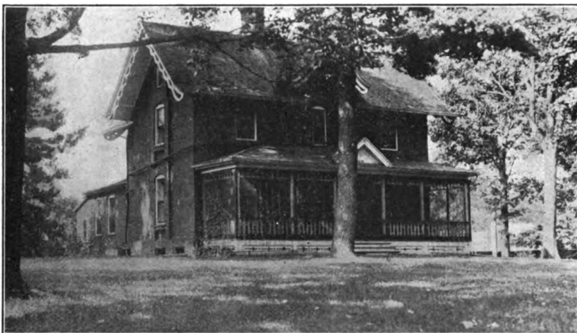
Looking north. Dwelling built in 1857, kitchen and porch added much later; now, 1913, occupied by Dean Shaw. Faculty row No. 5.
